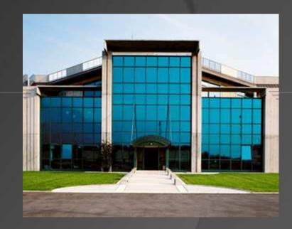
Insulating Glass Unit incorporating coated solar control glass
